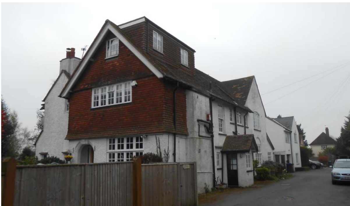
Figure 4. Front elevation of 2-3 Barrowsfield
